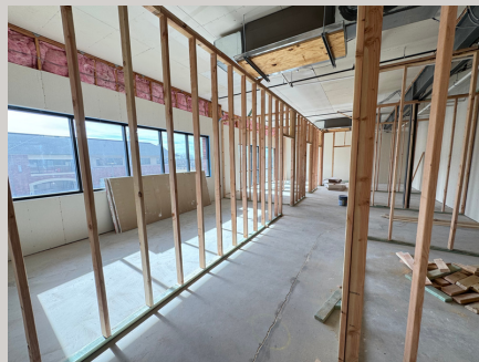
Office Build-out (in progress)
